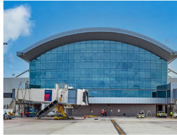
A two-story expanse of windows gives passengers access to an abundance of natural light and views.
